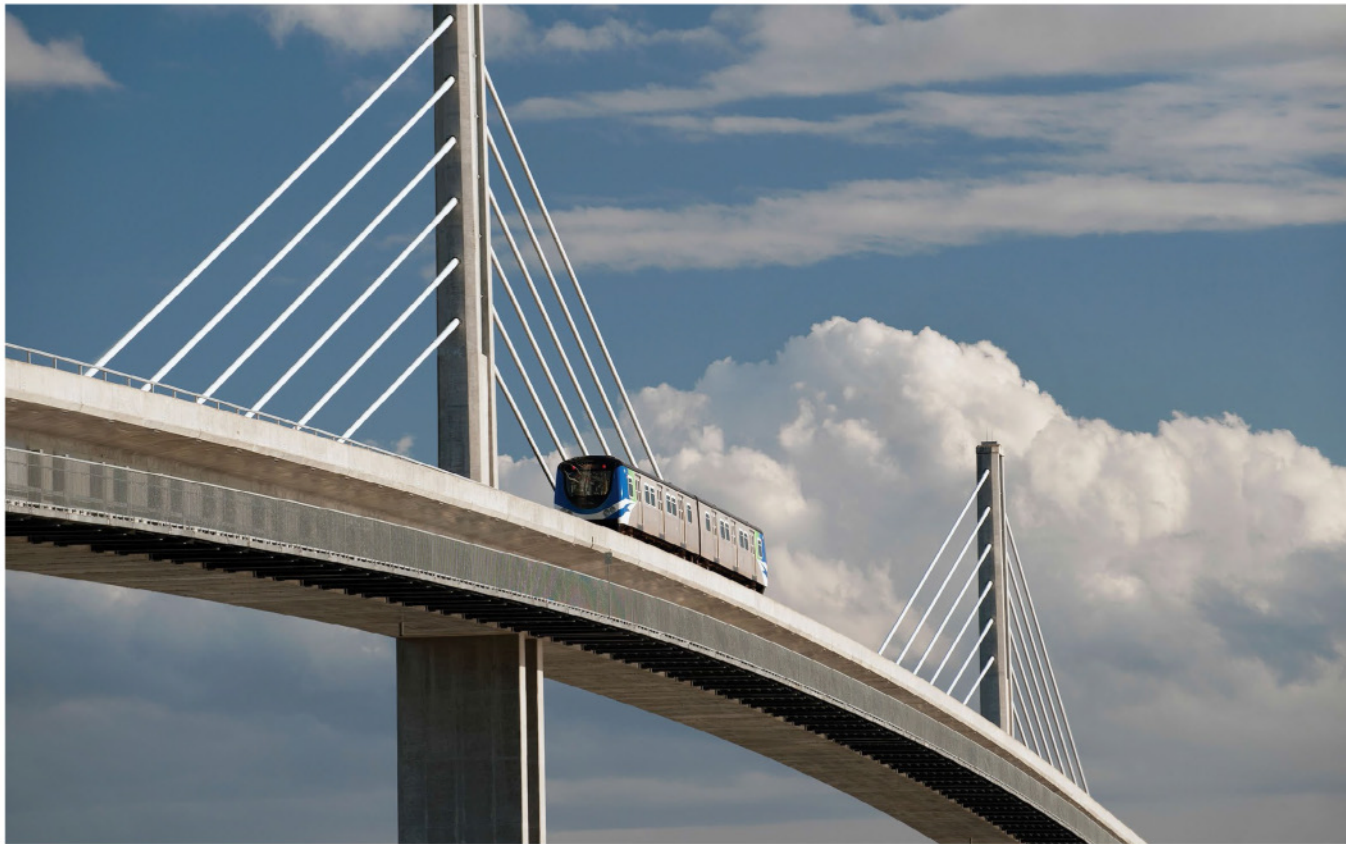
BBGI Global Infrastructure has invested in the Canada Line SkyTrain in Vancouver
